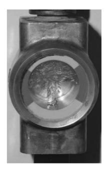
Fig. 4-23 Bubbles in the sight glass due to refrigerant shortage
